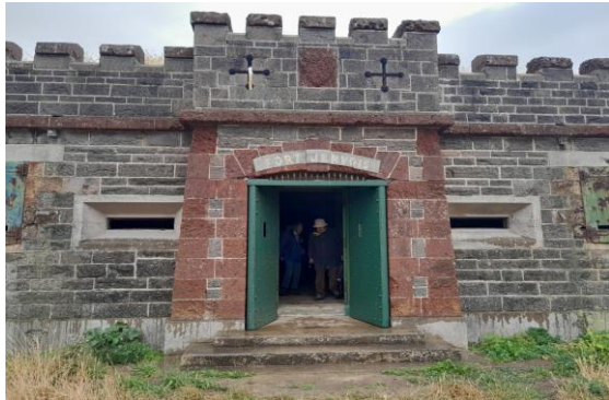
Entrance to the tunnels
