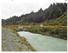
The Geo/Bot bus trip this month was to the Rangitata Diversion Race which takes water from the river for irrigation. It was built in the 1930s, dug by hand for 42miles at a gravity fed rate of 1foot of drop for every mile. It is 12ft deep and 12ft wide, so an enormous task but still working well to this day.
